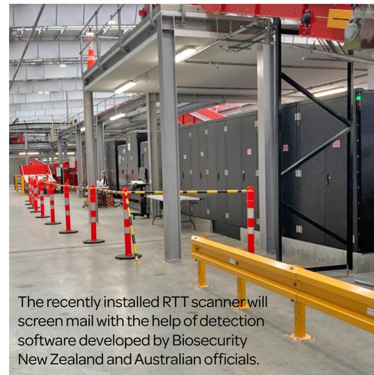
The recently installed RTT scanner will screen mail with the help of detection software developed by Biosecurity New Zealand and Australian officials.
