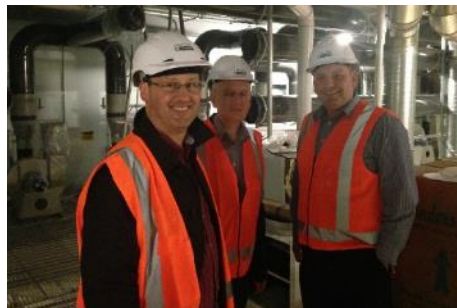
MPI Project Manager Mike Hannaway, Project Director Dr. Joseph O'Keefe, and FCC Project Manager Chris Edwards visit a lab currently under construction
