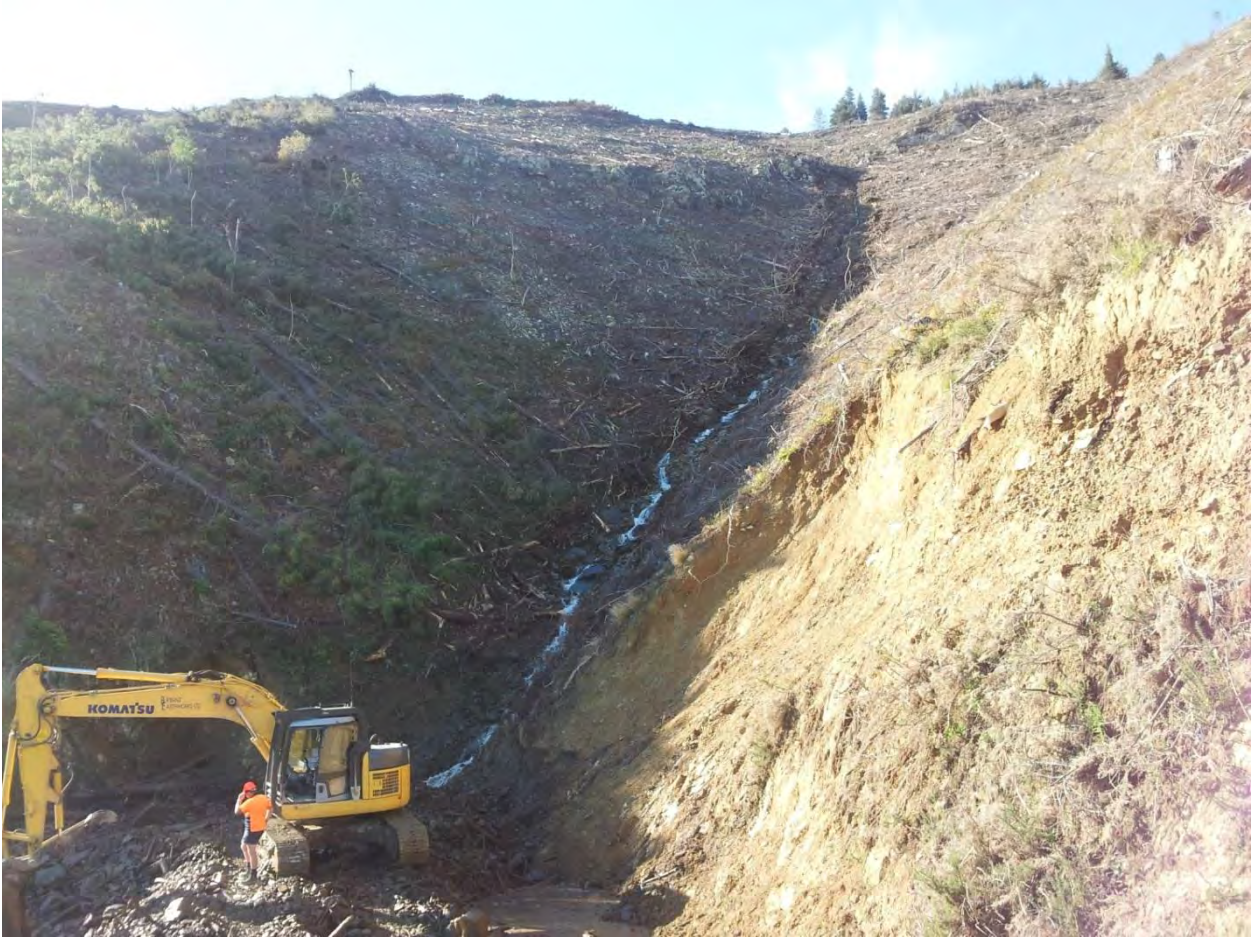
Figure 3: Slope failure post forest harvest. Note proximity to water body and slip material blocking flow leading to direct transport of fine sediment into estuary.
