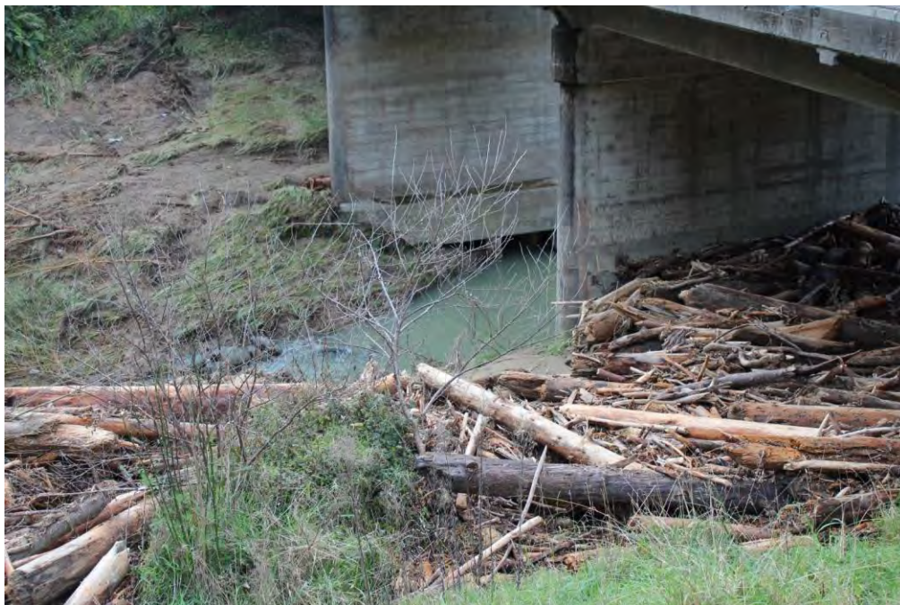
Damage to infrastructure – this is one of 5 SH2 bridges over the Maraetaha River – farm culverts, bridges and fences are also frequently affected by forestry slash mobilisation from slopes.
