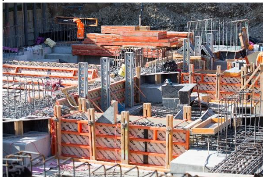
Boxing up the steel in preparation for pouring concrete.
