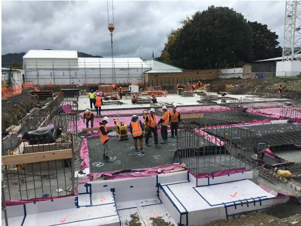
The concrete in the background of this image will form the basement floor. The next stages of construction include completing the concreting in this area, forming the base isolator plinths, and installing base isolators.
