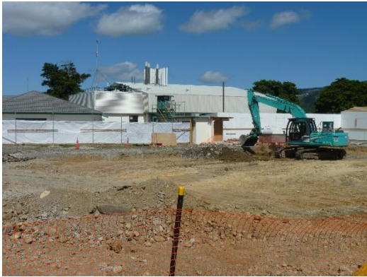
A digger excavates the site before the foundations can be laid. The existing high-containment laboratory is visible in the background.
