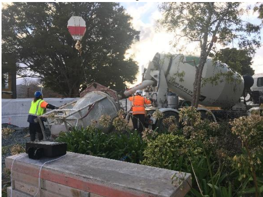
Contractors fill the concrete skip for the next load.
