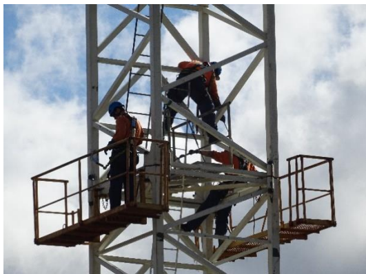
Contractors work to assemble the crane on site.
