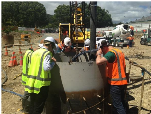
MPI engineers watch the first concrete anchor being poured.
