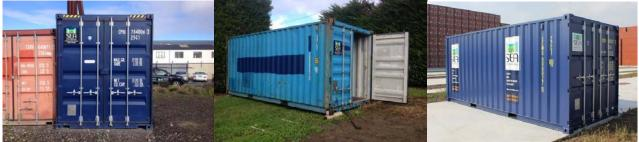
Placed on gravel and <1m spacing Placed on grass and too close to trees Too close (<1m) to vegetation and soil
