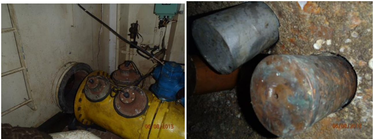
Figure 63. External (left) and internal (right) views of MGPS anodes fitted to pipework just inboard of sea chest.
