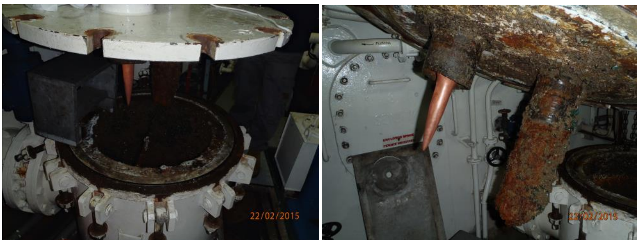
Figure 65. MGPS anodes fitted to the lid of a high intake strainer box.
