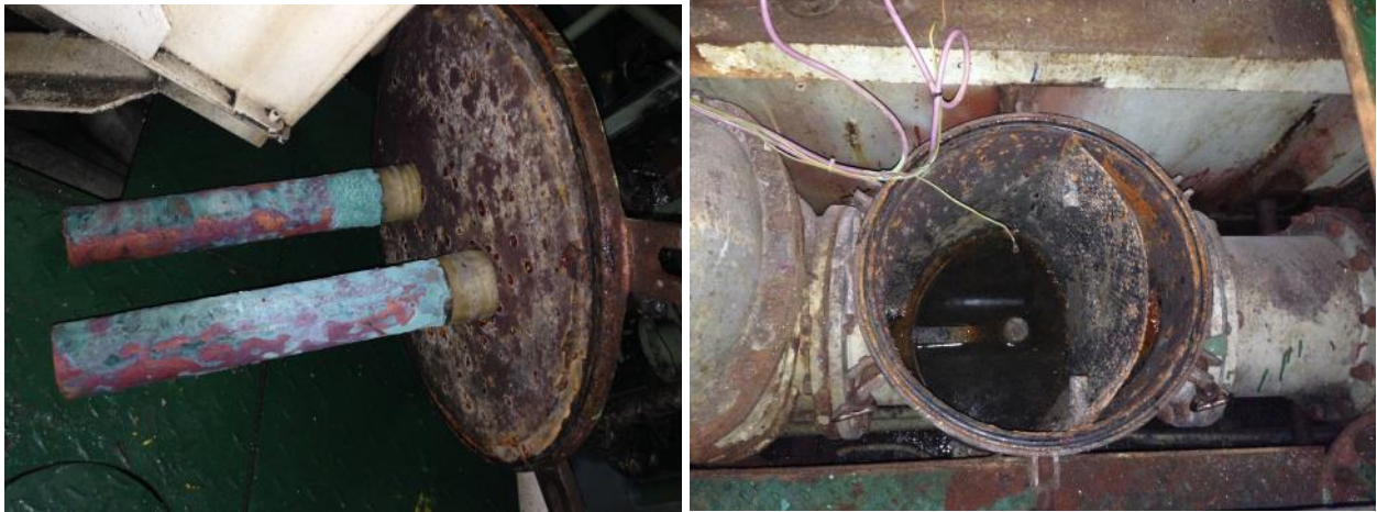
Figure 64. MGPS anodes fitted to the lid of a seawater intake strainer box.
