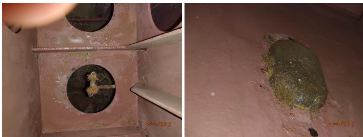
Figure 33. SPC1-coated sea chest at 23 months with macrofouling only on projections and unpainted anodes.
