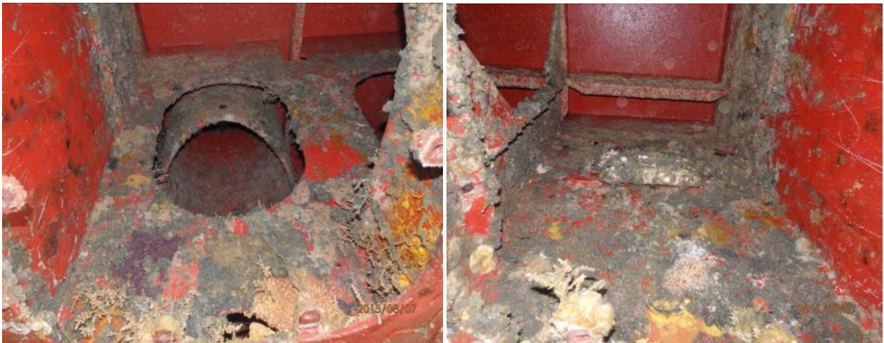
Figure 37. FRC-coated sea chest at 40 months. Some walls have almost no attached macrofouling while others are extensively covered.
