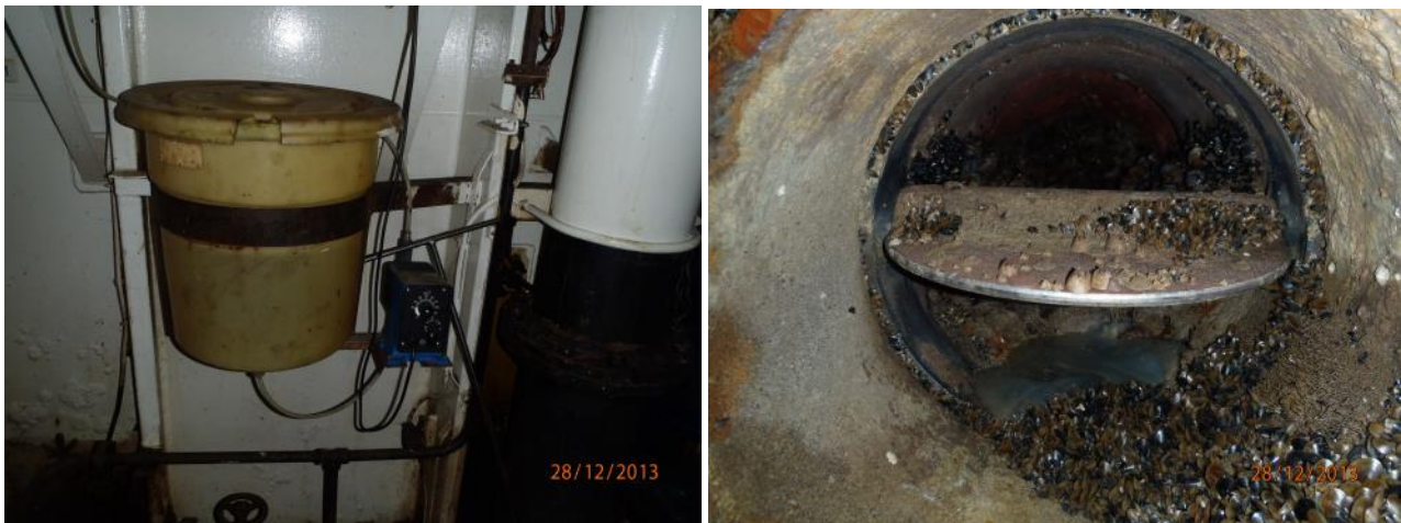
Figure 68. Chemical reservoir for dosing and hull isolation valve in the chemically treated system.
