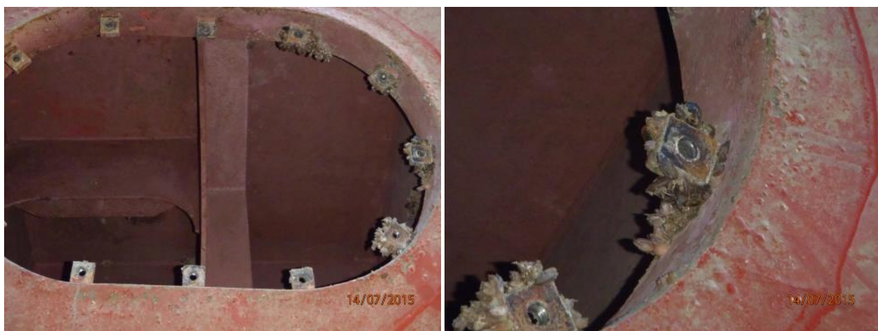
Figure 34. Another SPC1-coated sea chest on the same vessel as in Figure 33 showing macrofouling restricted to paint imperfections on grate attachment lugs.
