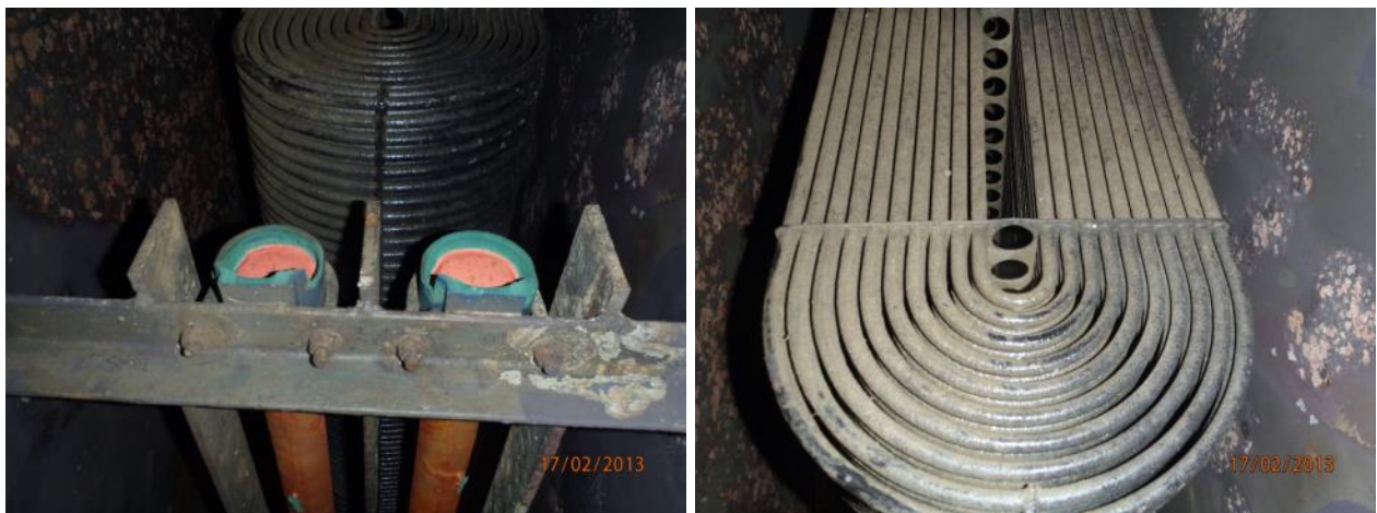
Figure 61. Cleaned box cooler with copper anodic MGPS.
