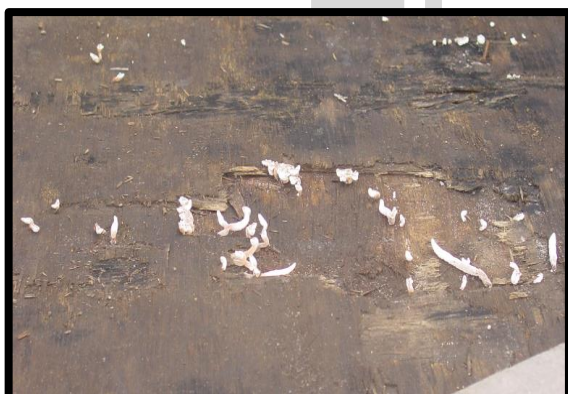
Check rotten wood for insect infestation, larvae and maggots. Rotten wooden will need to be treated or removed.
