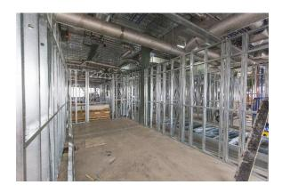
Internal steel wall frames are being installed giving the first physical view of how the laboratory floor space will look.
