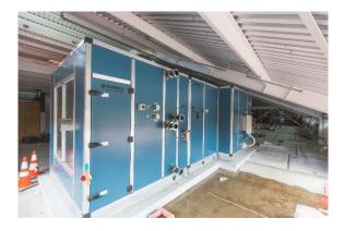
Large pieces of plant such as air handlers and pumps are arriving on site and being installed on custom made plinths on the upper floors.
