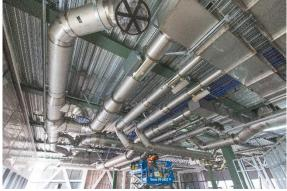
Complex ductwork and pipework is being connected to the various plant, suspended in what will eventually become the interfloor spaces.
