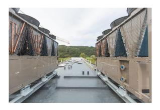
Given the large spaces and exacting requirements of the new laboratory the three machines are both grunty and robust, with the 8 fans on each chiller being able to shift more than a 20ft shipping container of air every second. Control of environmental conditions within the laboratory spaces is essential in maintaining containment.
