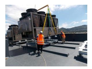
The chillers will provide both cooling and heating to the new laboratory, achieved by extracting energy from the outside air using vapour compression much like your fridge at home. This energy is used to heat or cool water which is then pumped into the building.
