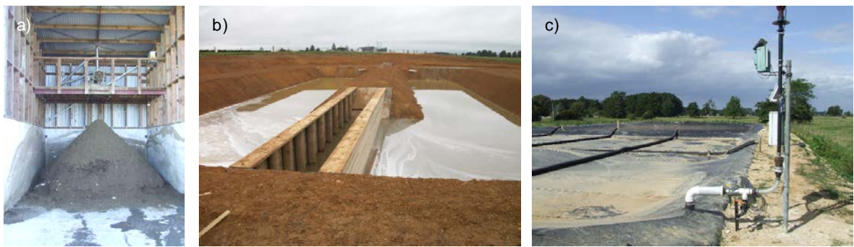
Figure 3: Typical effluent pre-treatment systems in NZ, employed prior to deferred-irrigation storage ponds : a) mechanical screw press separator, b) weeping-wall system, c) covered anaerobic pond. (Photos a, c): S. Heubeck; b): John Scandrett, Dairy Green.)
