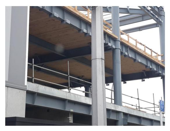
Notice that this mid-rise building, constructed in steel, shows Cross Laminated Timber (CLT) being used for the flooring instead of concrete. The CLT was supplied by Red Stag Investments, the industry partner in the Mid Rise Wood Construction programme. This building is in Rotorua, New Zealand's first city to adopt a "Wood First" policy.
