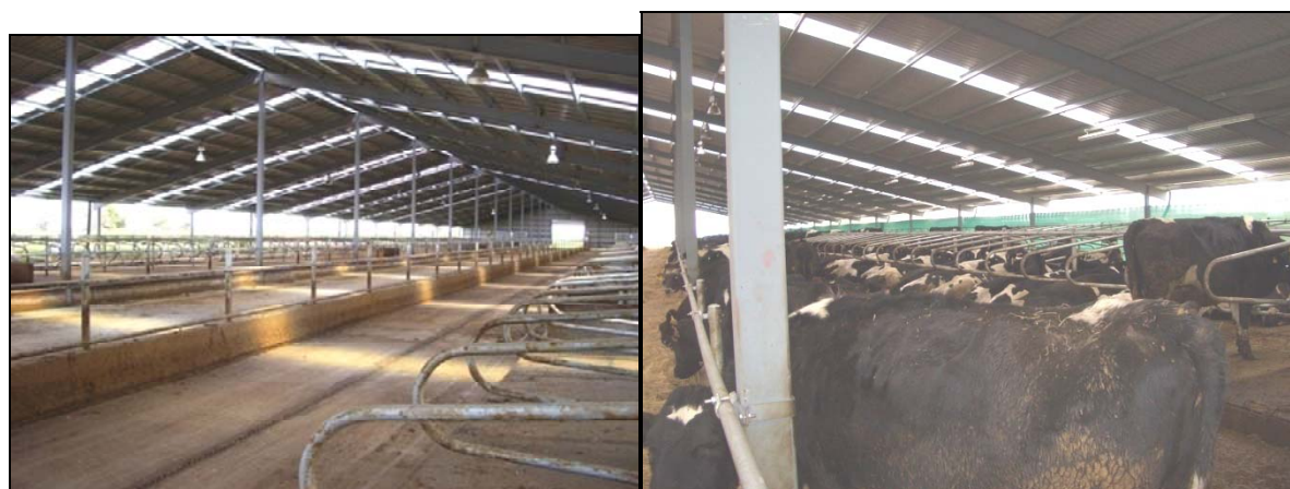
Figure 11: left: free-stall barn for 500 cows, configuration with central feed alley, solid concrete floor with effluent scraper, three rows of stalls on one side and two on the other; right – cows feeding and resting in a free-stall barn (photos: Gwyneth Verkerk).
