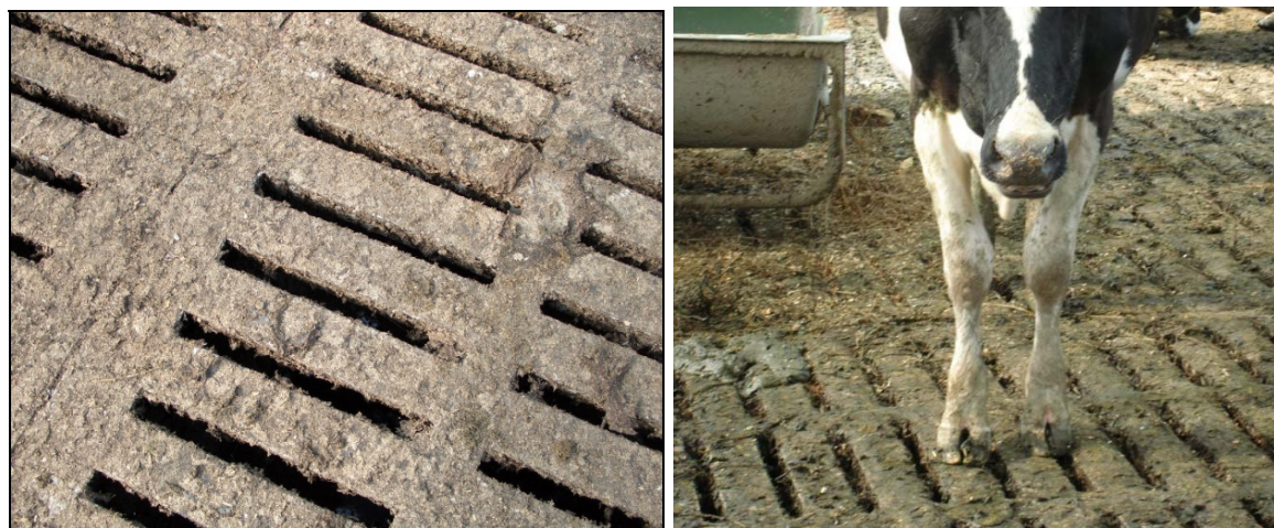
Figure 7: Left – slatted floor configuration used in Herd Home ® shelters; right – cow foot size relative to slat size in Herd Home ™ (photos: Tom Pow, Herd Homes ™ Ltd)
