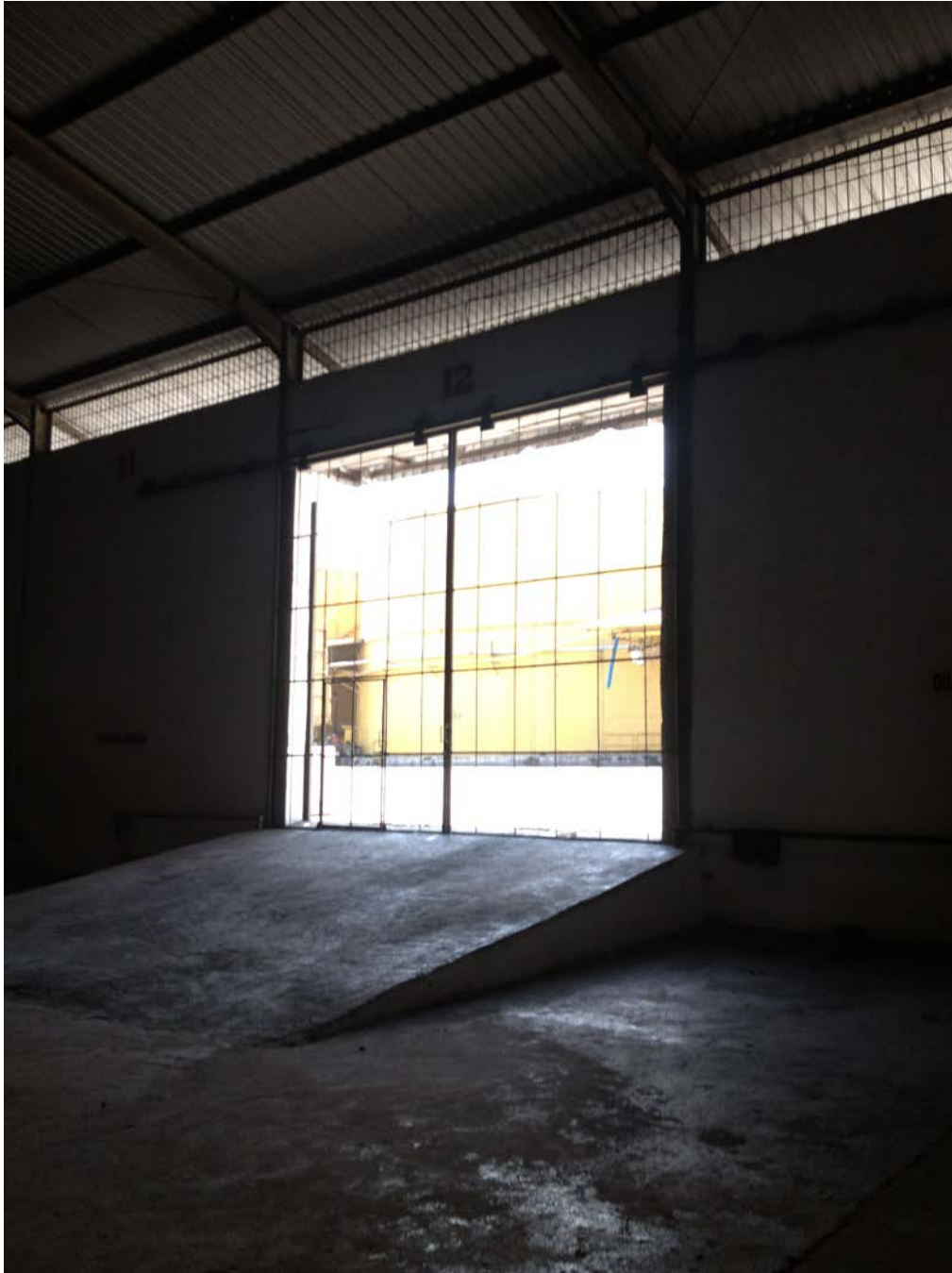
FIGURE 22: NETTING AT DOORS AND GAPS IN PKE STORAGE WAREHOUSE
