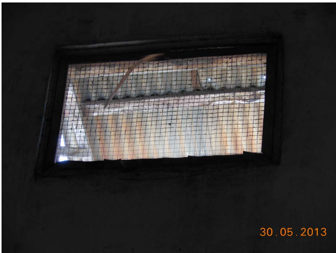
FIGURE 21: NETTING ON VENTS WITHIN PKE STORAGE FACILITY
