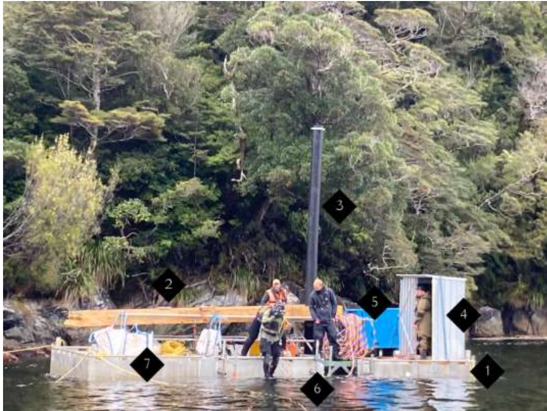
Figure 3: Primary work platform for suction dredge removal trials: 1) Non-powered barge attached moored using ropes and anchors; 2) Plywood biomass sorting table; 3) 6 m dropper pipe. Picture fully raised but lowered into the water column during operation; 4) Dive supervisor station including SSBA air supply and communications; 5) Low-pressure compressor to supply airlift system; 6) Dive platform. 7) Fades for biomass collection.
