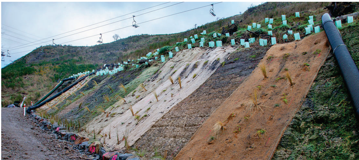
Figure 1: Geotextile products being trialled in Banks Peninsula by EOS Ecology (McMurtrie, 2020).
