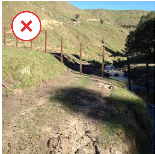
Right: This slash trap is a non-engineered structure in a large catchment (>1000 hectares). It will likely fail in a significant event because it won't withstand the volume of debris and water that such a large catchment could generate and deliver.
