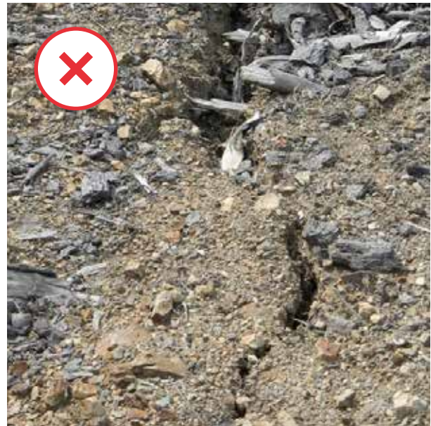
Right: Tension cracks on the edges of landings can indicate minor fill settling or they can be the precursor of a potential failure. Relocate slash from the landing edge onto the hard surface before the crack. Install water controls to stop water getting into the crack and further lubricating that structural weakness.
