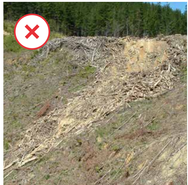
Right: Poor landing drainage collapsed the landing fill.
