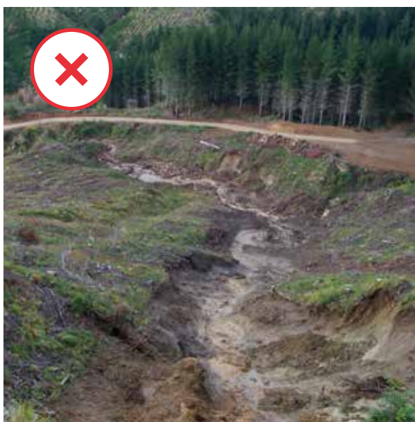
Right: Landing failures often generate debris flow and landslides. The image looks 400m down an eroded gully created from this landing failure.
