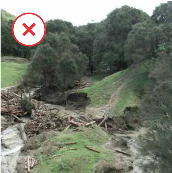
Left: The slash trap was designed to direct slash onto the floodplain. Instead, it failed due to a weak anchor.
