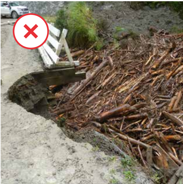
Left: Bridges are usually sited at the narrowest waterway width. Constricted waterway sections may also bottleneck or accumulate slash.
