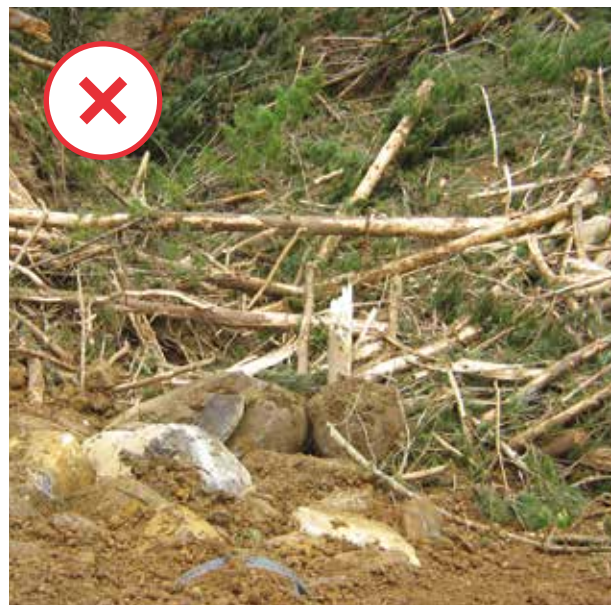
A slash choked culvert is an example of poor slash management practice near a waterway.
