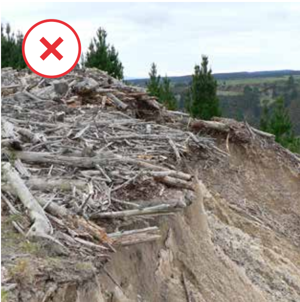
Left: This landing was not rehabilitated and had a bird's nest failure four years after harvest.
