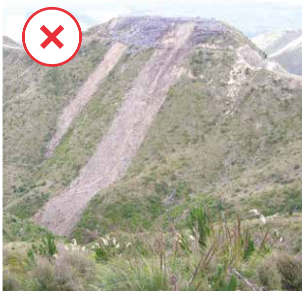
Inadequate slash management and water control caused the landing failure.
