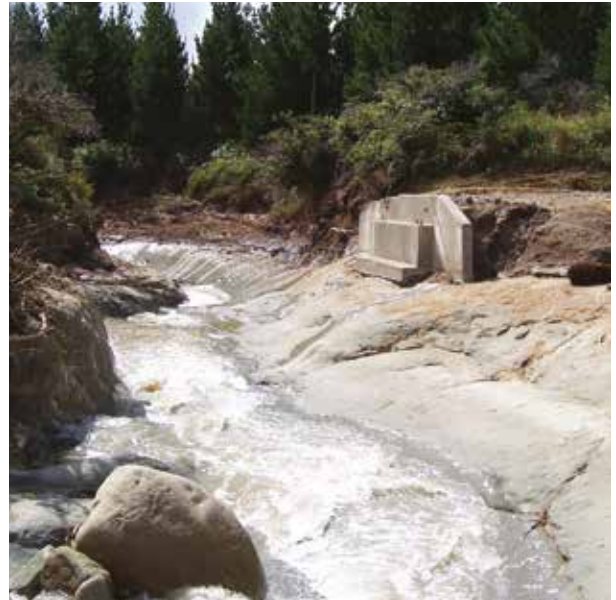
Right: The aftermath of a debris dam/flood that started several kilometres upstream. The bridge deck was never found. The waterway's bed and banks were polished.
