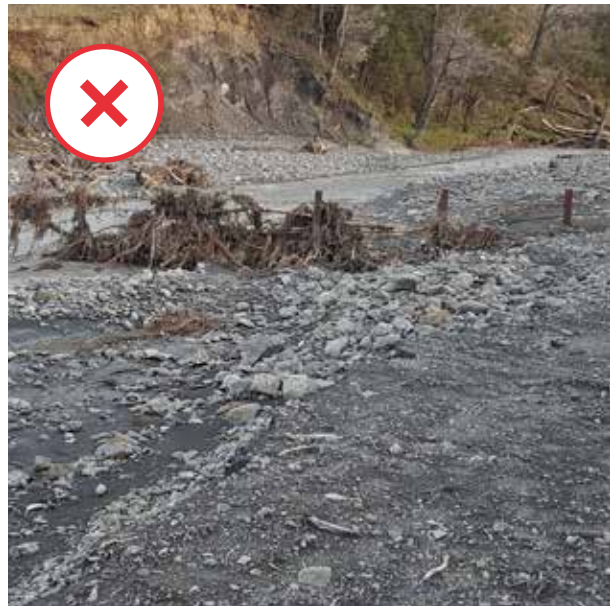
Right: The slash trap should not be constructed across a major waterway.
