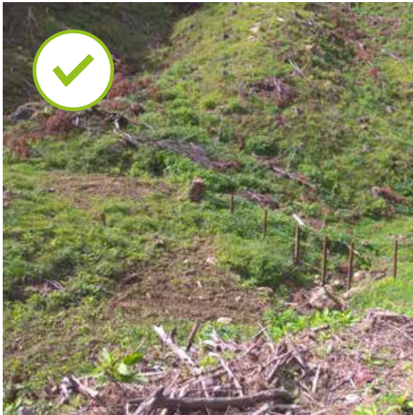
A railway iron/cable debris trap anchored by stumps in a catchment <20 hectare.
