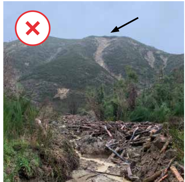
Right: This debris flow was initiated at the landing (black arrow). Stormwater was being drained into a pocket bench that failed.
