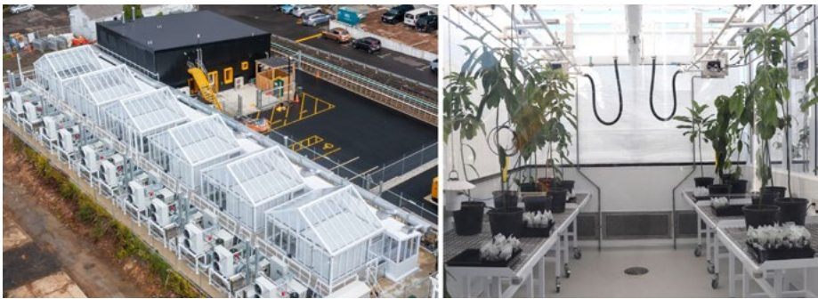
Figure 3: An aerial view of the new level 3B post-entry quarantine greenhouse facility in Mount Albert, Auckland (left); and plants in one of the 12 units that were used for biological commissioning (right)
