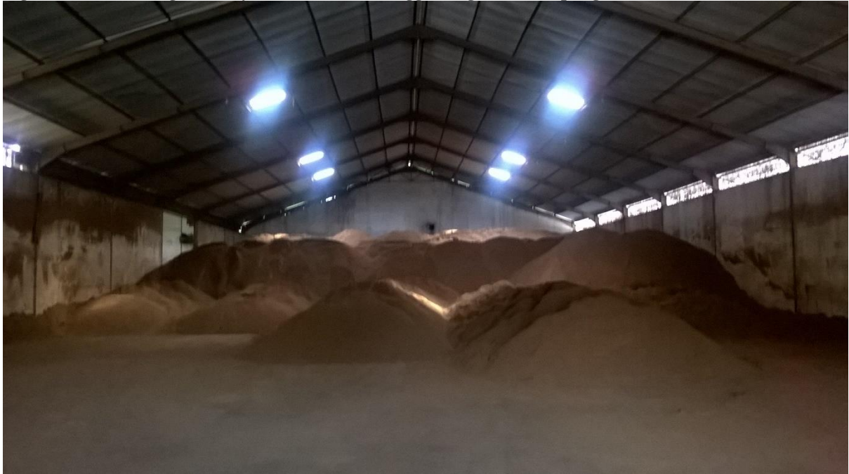
Figure 4: PKE Storage Facility at PT. Kurnia Tunggal Nugraha, Lampung
