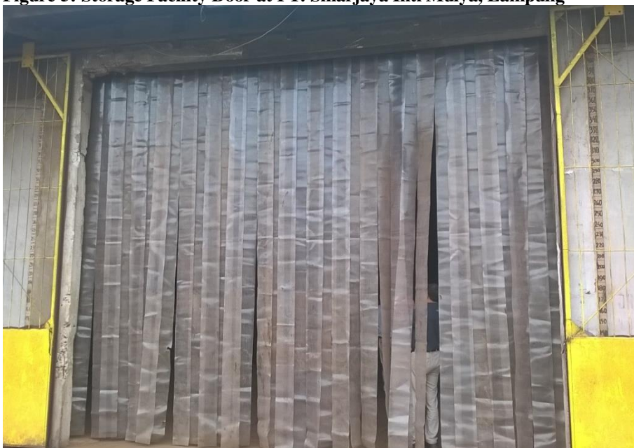
Figure 5: Storage Facility Door at PT. Sinarjaya Intl Mulya, Lampung
