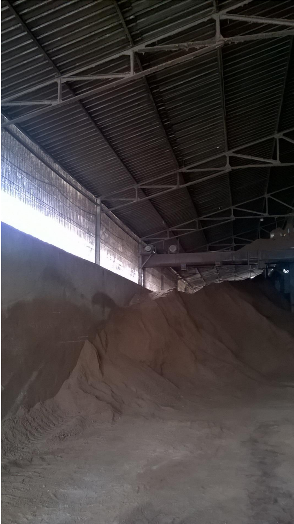
Figure 12: Storage and netting at a PKE Storage facility
